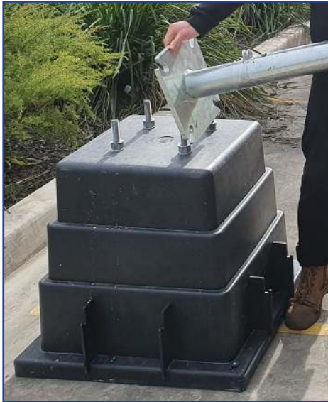
Fig. 2.3a Mounting pole onto concrete base
