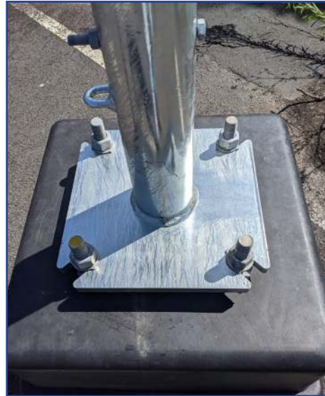
Fig. 2.3b Pole fixed onto on concrete base
